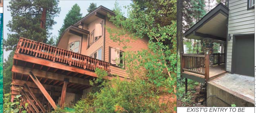
NORTHEAST VIEW OF EXIST'G HOUSE
