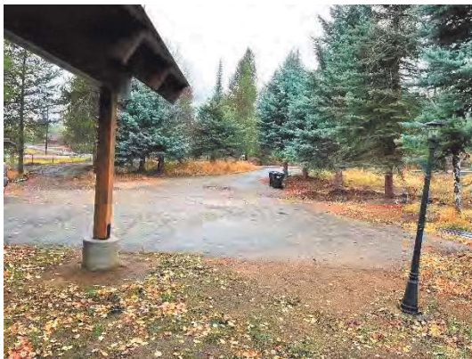
main house parking area
